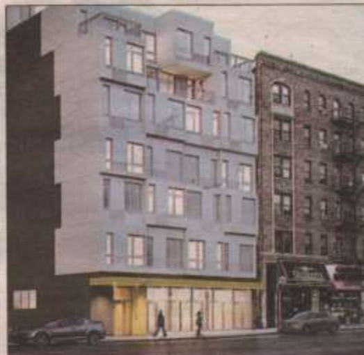
The Stack is made up of 56 modules.
