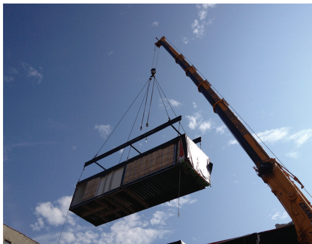
A module is lowered onto The Stack
